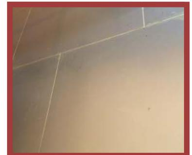
7. Start the second row from where the first ended to give the boards a staggered joint. Follow the same procedure until the wall is completed. Ensuring the first board is flush and square will make the rest of the installation easier.
