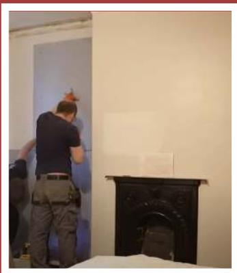
3. SoundBoard3 is supplied in standard sheets (1.2m x 1.2m) which are fixed directly to the wall.
