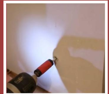
6. Once the first board is in position, apply the second board butting up tightly to the previous board and continue. (Only seal between boards if any gaps appear).
