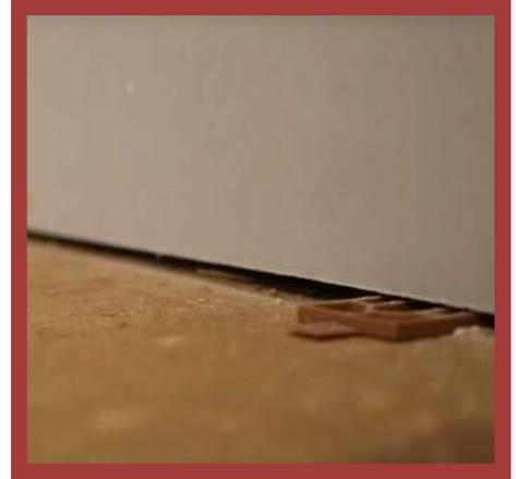
5. Fix the boards directly to the wall by drilling 9 holes and fixings per board (50mm into the original wall) then fix with Hammer screw fixings.
